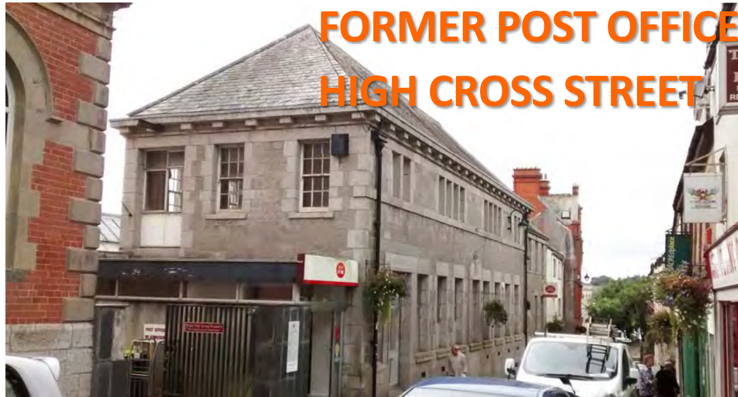
Above: View of High Cross Street showing the positive contribution the old stone building gives to the Conservation Area
