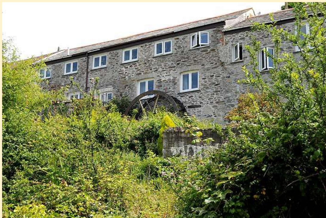
Old mill on Bodmin Road. Located on the route of the leat from Menacuddle, which powered its waterwheel.
