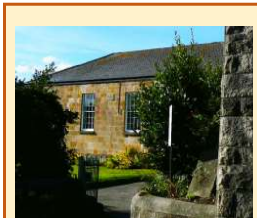
The warm colour of Pentewan stone on the Quaker Meeting House contrasts with the Carn Grey granite on the retaining wall to the station.
