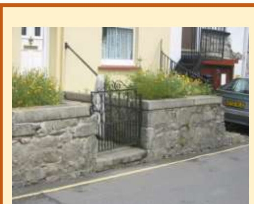
Low stone walls with dressed granite copings bring character and enclosure to the street.
