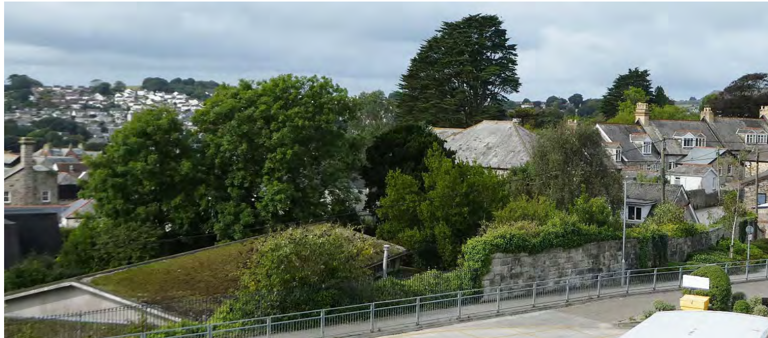
Above: The higher view from the railway line across the site.
